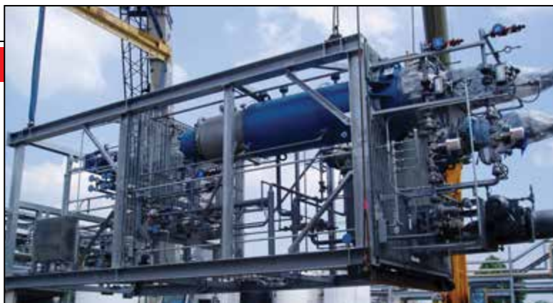
FIGURE 1. The modular process-system-design approach was utilized for this evaporator system, shown here being lifted from the truck and righted for plant installation. Modular construction includes mounting all process equipment on a structural steel frame, fabricating all interconnecting process and utility piping and installing all instruments on the module and wiring the instruments to a junction box or control panel. A modular design/build firm provides single-source responsibility for the modular process system
