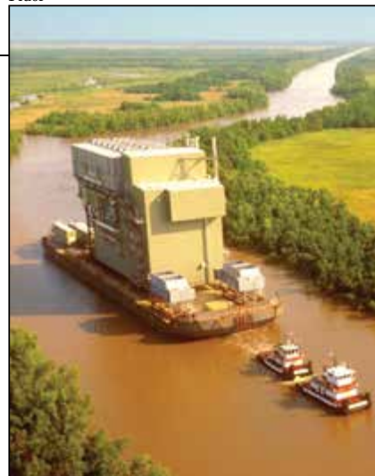
FIGURE 4. Due to the remoteness, offshore platforms are almost exclusively built on a modular basis in the shipyard and then floated out to the site
